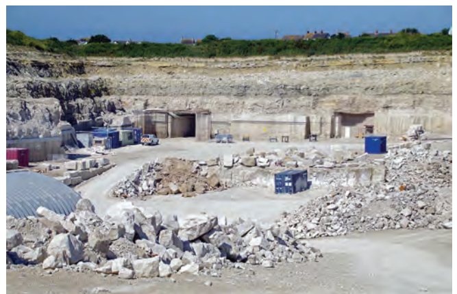
Looking west across the Perryfield quarry floor. The left-hand portal is the working adit, the right-hand a blind portal to be used in the future as an exit
